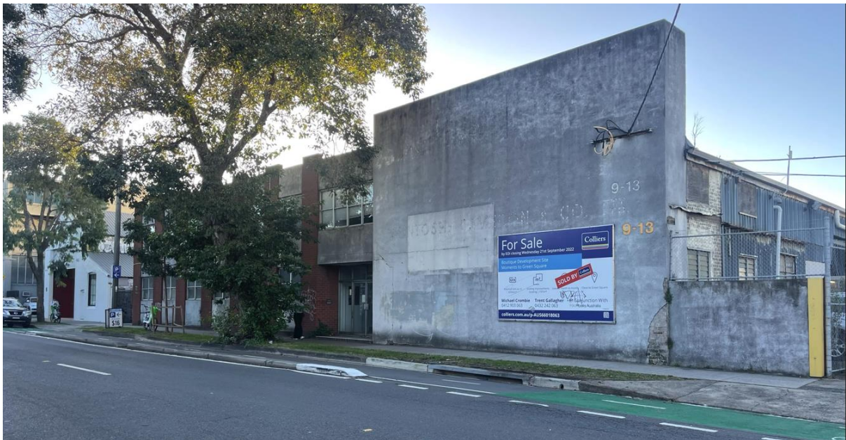
Figure 10: Existing warehouse development opposite the site at 9-13 Bourke Road
