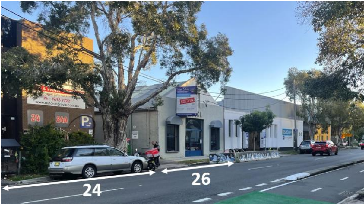
Figure 7: View looking west down Bourke Road showing 24 and 26 Bourke Road and 28-32 Bourke Road beyond
